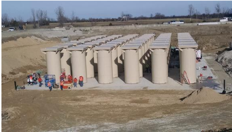
48 CECs placed on Support Foundation Pad
