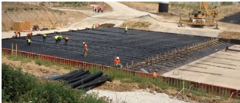
HI-STORM UMAX Support Foundation Pad
