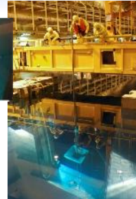
Loading a basket in a dry storage cask
