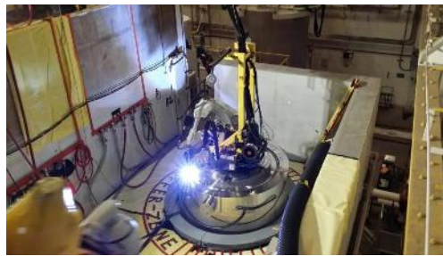
Robotic Welding on First Fully Loaded Fuel Canister
