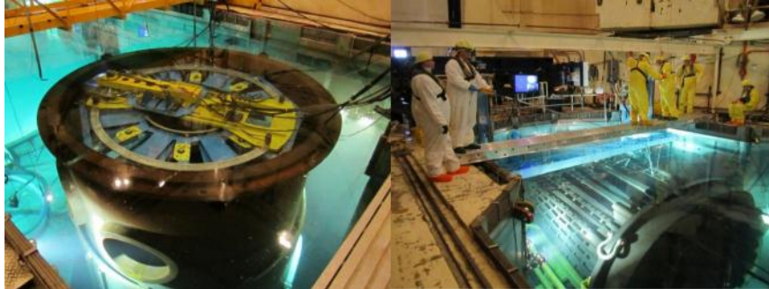
Cutting on Upper internals and lower core barrel from Unit-2
