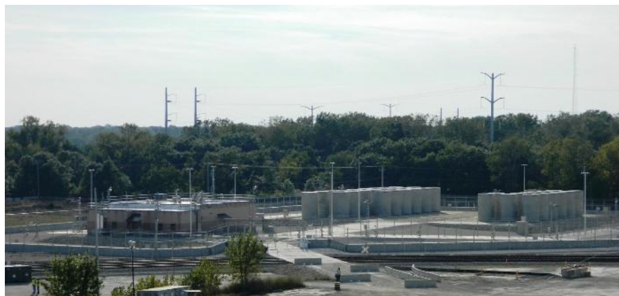
ISFSI on 9-9-14 with 37 of 61 Dry Storage Casks in Place Spent Fuel Loading is 100% Complete as of 8 Jan 2015!
