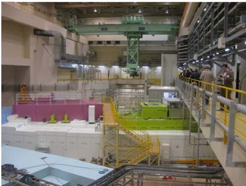
This picture was taken inside the Japan Proton Accelerator Research Complex (J-PARC). Workshop attendees toured the facility on the last day of the workshop
